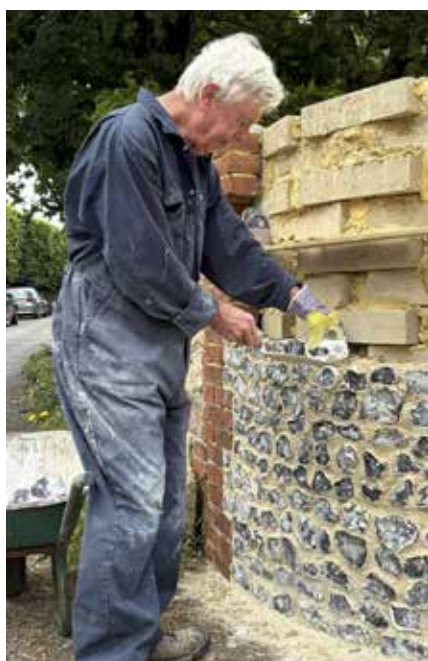
Peter Henderson rebuilds a traditional flint wall at The White House, Amberley
