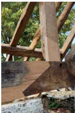
Joint repairs
